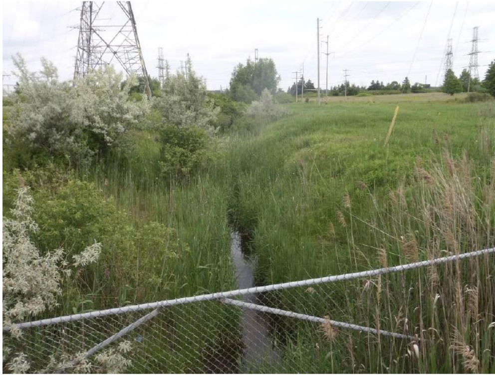
Photo 3 – Elliot Laidlaw Drain (Site No. 19- 351/c): At culvert facing upstream (north)
